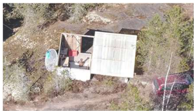
Sliding roof observatory
